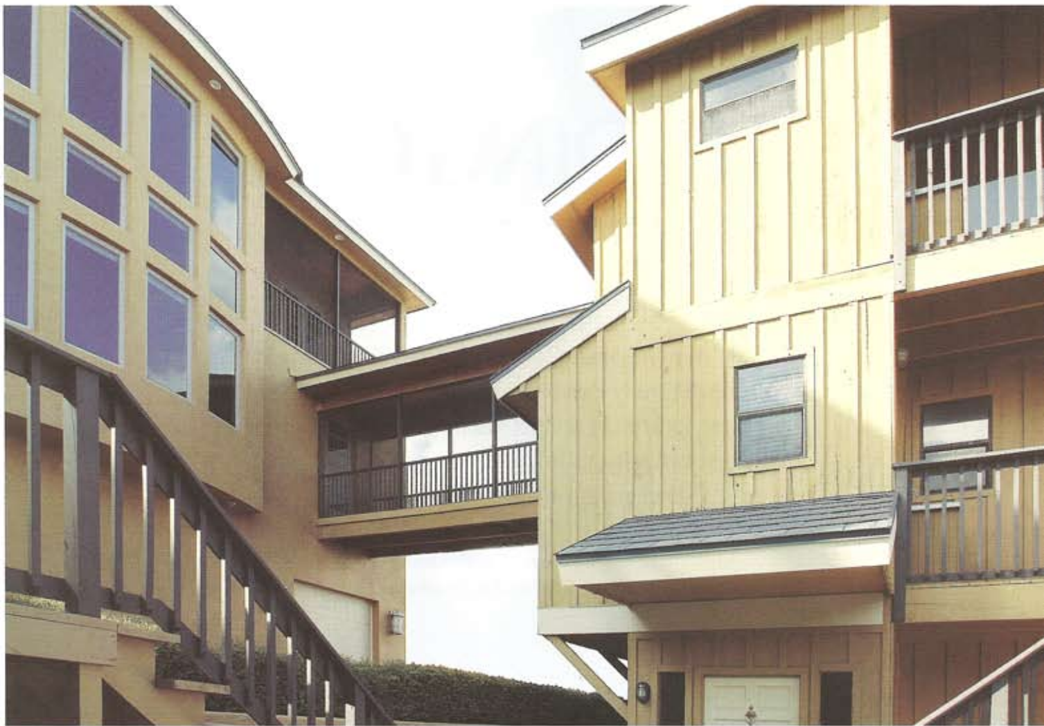
Above: The rear exterior of this Cocoa home, with architecture by Tony Mazza, offers a screened-in walkway, connecting to an adjacent three-story home with wood paneling and sharp architecture. Previous pages: Fine detailing is prevalent throughout this Jackson Kirschner Architects' French country-inspired Lansing Island residence, which required extensive historical research to design.
